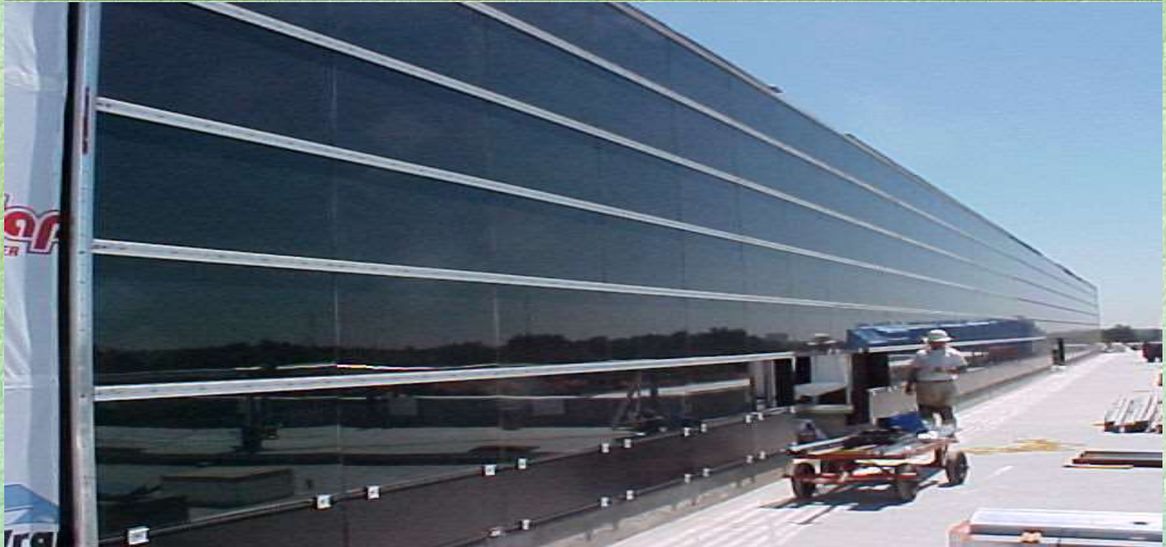
East End Office Complex 24 kW BIPV Curtain Wall
